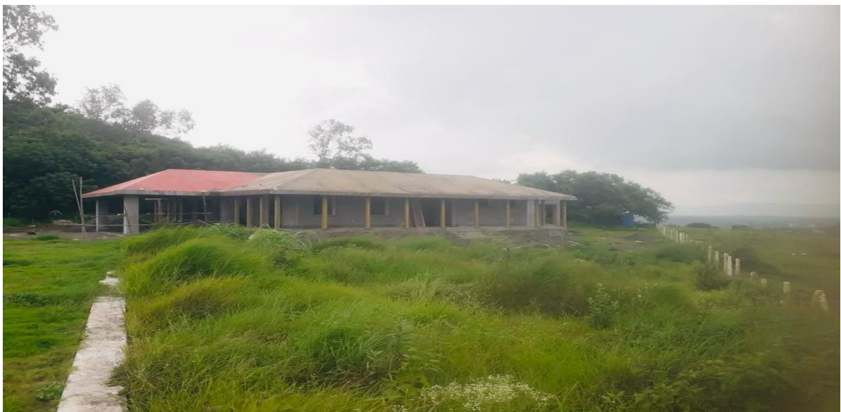
COMPLETION OF RCC, BRICKWORKS AND PLASTER
